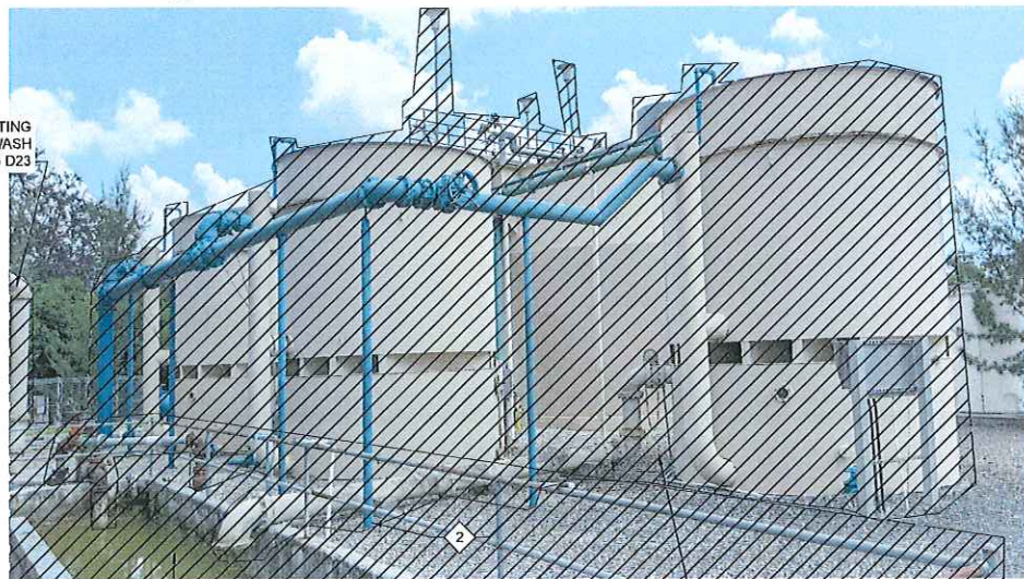
DEMOLISH EXISTING FILTER BACKWASH RETURN BASIN, SEE DRAWING D24
