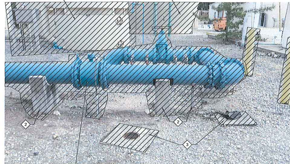
DEMOLISH AND DISPOSE OF ABOVE GRADE INJECTION POINT 2 PIPING AND APPURTENANCES. SEE GENERAL NOTES.
