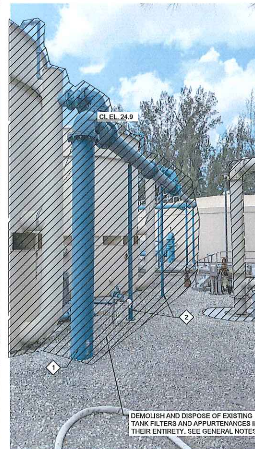
AU PHOTO FILE: TANK FILTERS 1-4
