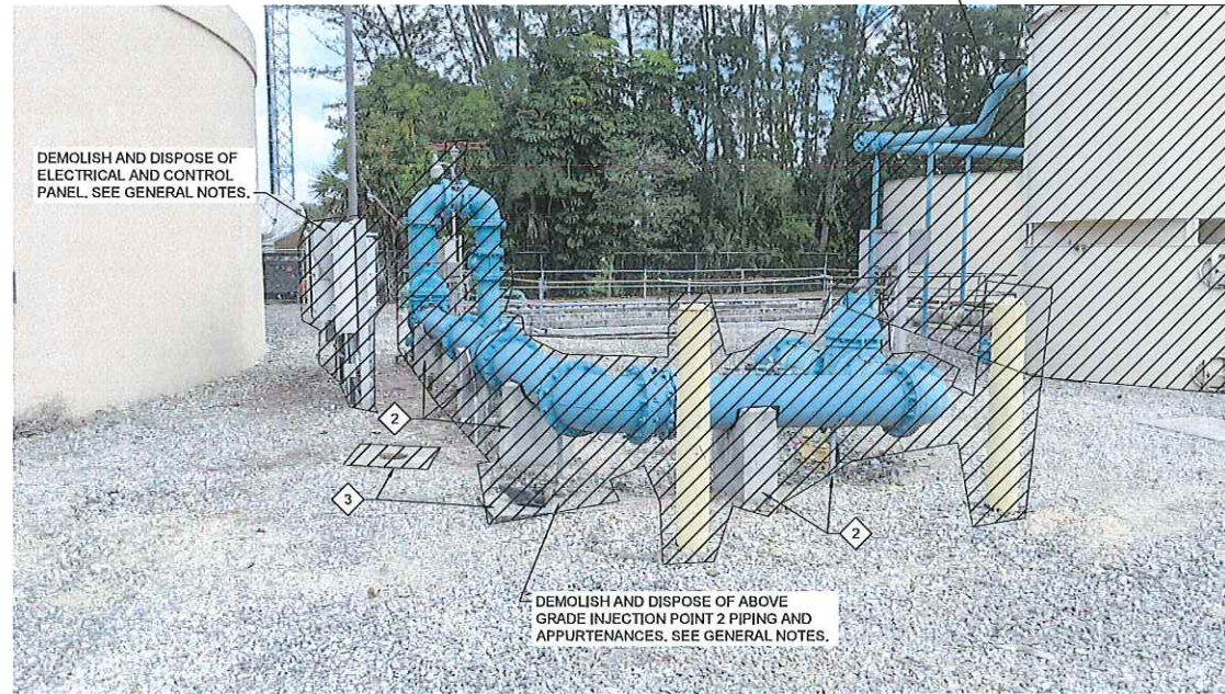
BO PHOTO FILE: INJECTION POINT #2-2
