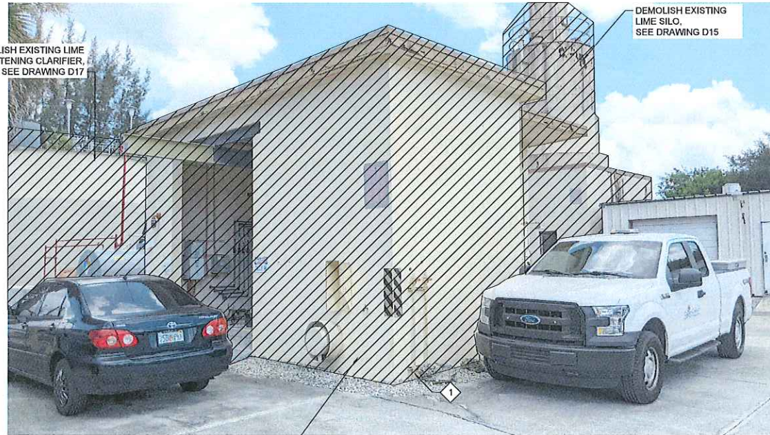
DEMOLISH AND DISPOSE OF CHLORINE STORAGE BUILDING AND ITS CONTENTS IN ENTIRETY, SEE GENERAL NOTES
