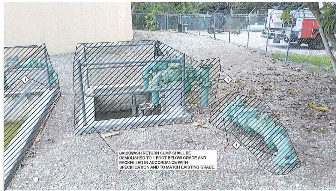
BL PHOTO FILE: BACKWASH RETURN BASIN - 3
