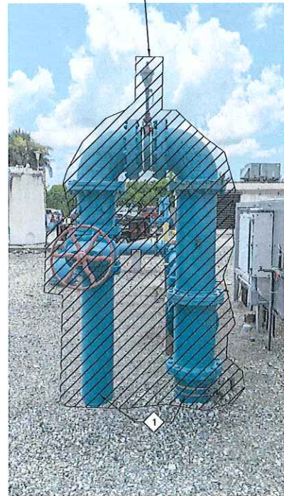
DEMOLISH AND DISPOSE OF ABOVE GRADE INJECTION POINT 2 PIPING AND APPURTENANCES. SEE GENERAL NOTES.
